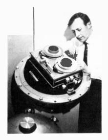
This underwater data centre – produced by GEC-Marconi – accepts inputs from almost any oceanographic instruments and records time-correlated data in computer retrieval form on magnetic tape.
